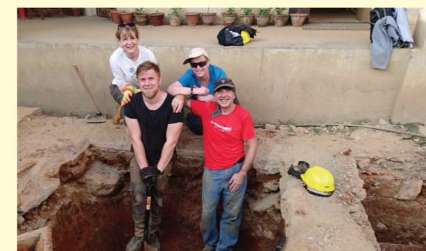
Digging the footings in Nepal
